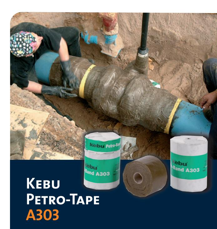
Cold-applied corrosion protection tape
