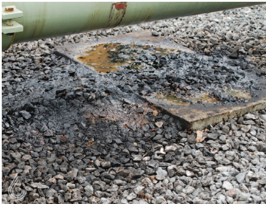
Before ESafe application: Hydrocarbon pipeline leak
